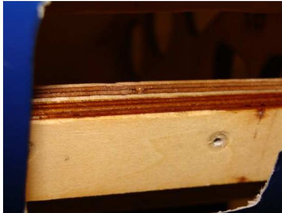
Fig. 6 - Example of block glued in place, screws removed. This area is now a full \frac{1}{2} " thick and stronger than factory built.
